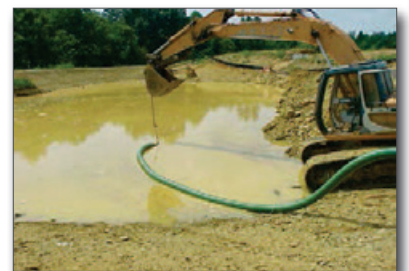
Figure 14. Sediment basin to be dewatered
