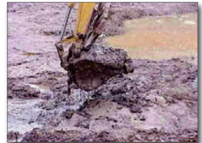
Figure 36. Removing stiffened sediment from a sediment basin
