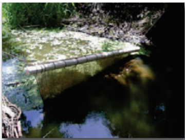
Figure 29. Particle curtain in a canal
