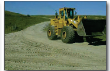
Figure 13. Road dust after applying polymer flocculant
