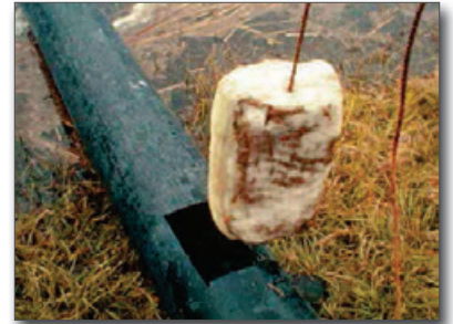
Figure 19. Polymer blocks inserted into pipes
