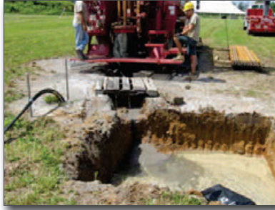
Figure 7. Drilling rig and settling pit
