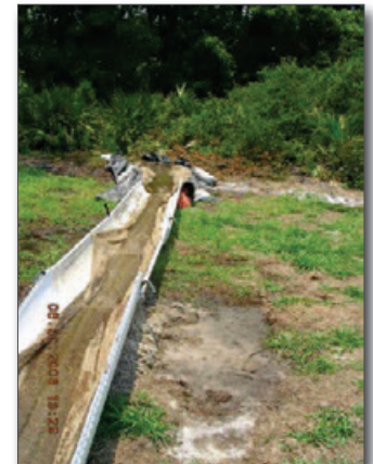
Figure 21. Split pipe with soft matting
