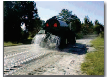
Figure 11. Water truck applying dissolved polymer flocculant
