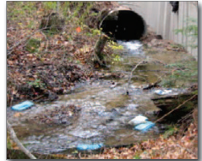
Figure 25. Six of the polymer blocks placed downstream
