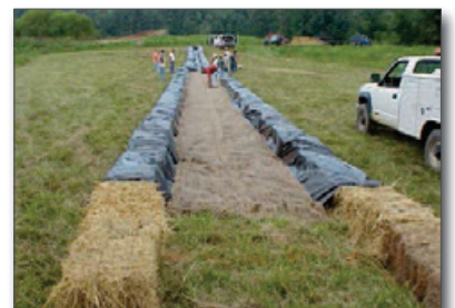
Figure 15. Lower portion of the treatment ditch
