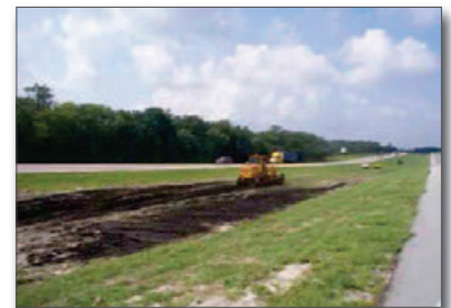
Figure 37. Recycling sediment along a highway
