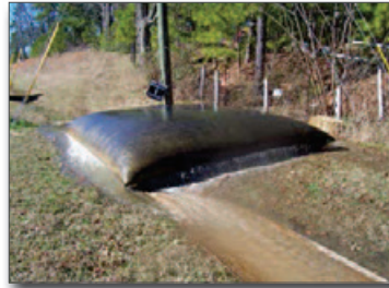
Figure 34. Sediment bag and its treatment ditch
