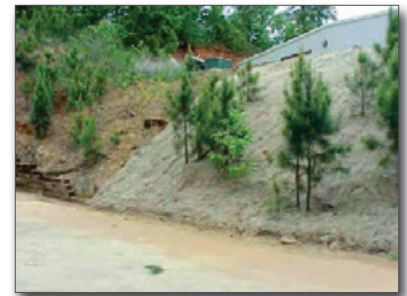
Figure 4. Slope covered with floc collection matting
