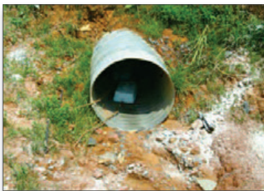
Figure 39. Polymer block in a construction site culvert
