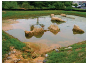
Figure 41. Same pond after BMPs were installed
