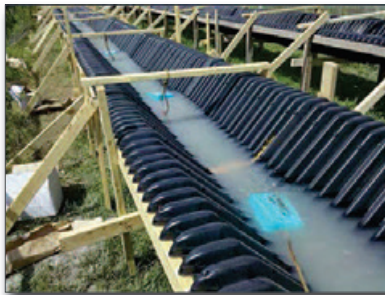
Figure 17. HDPE treatment ditch liner
