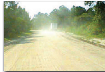
Figure 12. Road dust before applying polymer flocculant
