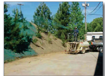
Figure 5. Hydroseeding the slope
